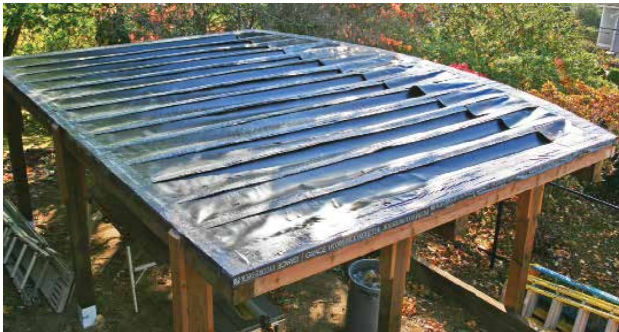
Figure 5. Self-adhering flashing protects the blocking and tops of joists from water damage. This freestanding deck also features an under-deck drainage system.
