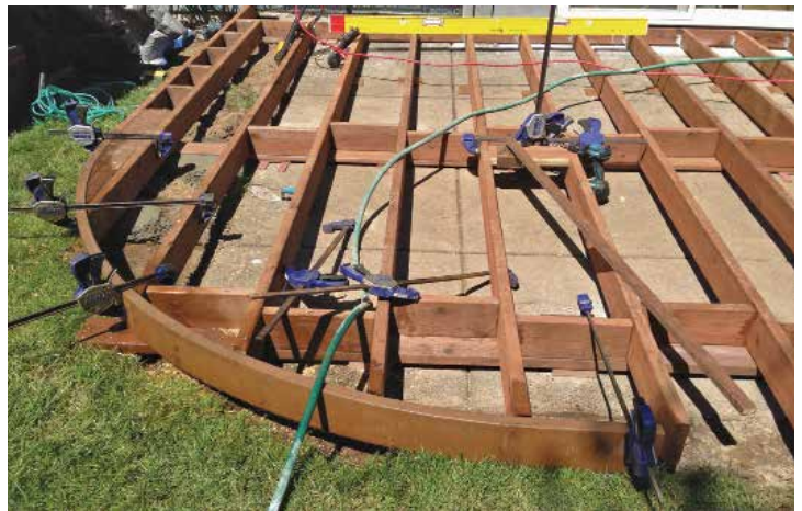
Figure 3. Rim joists are typically made up of 2-by composite or PVC decking stock ripped to match the width of the framing (above) and fastened to the ends of the joists with 3 1/2-inch-long structural screws (top right). Clamps are often needed to bend the rim joist around a tight radius (bottom right).
