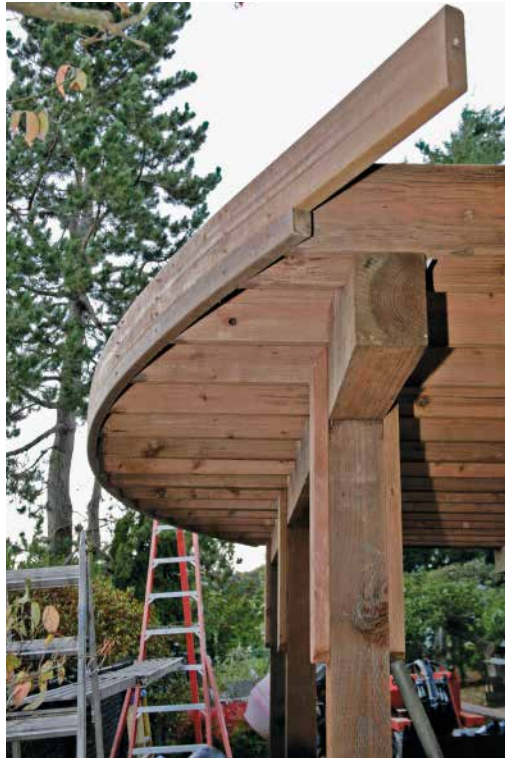
Figure 3. Rim joists are typically made up of 2-by composite or PVC decking stock ripped to match the width of the framing (above) and fastened to the ends of the joists with 3 1/2-inch-long structural screws (top right). Clamps are often needed to bend the rim joist around a tight radius (bottom right).
