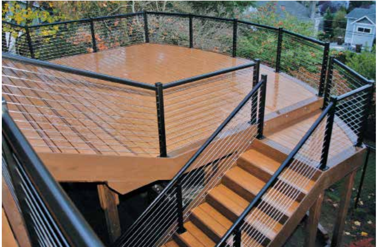
Figure 7. A faceted railing made up of short sections of straight rail looks fine on most curved decks (above). But when the curves are tight, some rail kits can be heat-formed to match (left).
